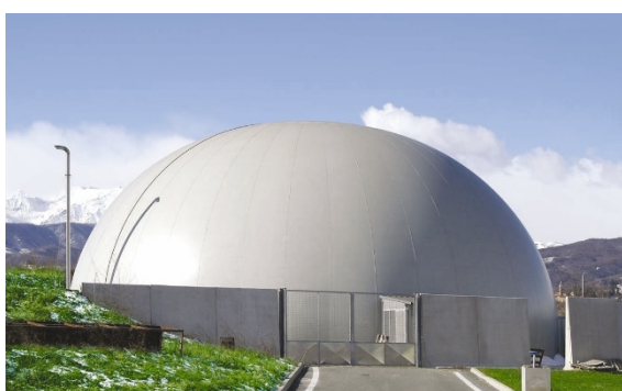
(3) Biogas Storage Tank
